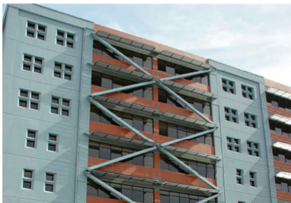
Structurally reinforced hospital, Ecuador (PAHO)
